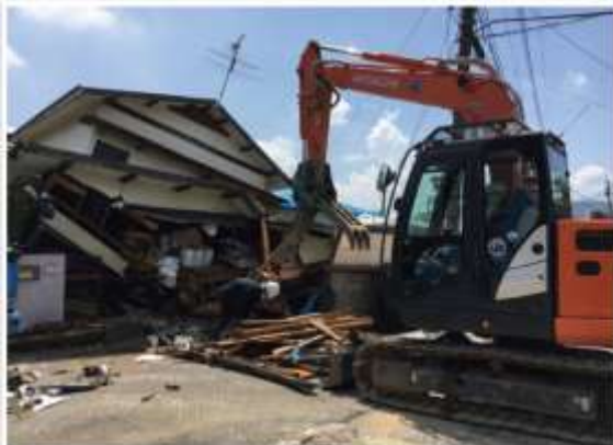
Dismantling and clearance of a collapsed house
