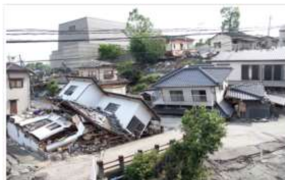
Damage from the Kumamoto Earthquakes in Mashiki Town
