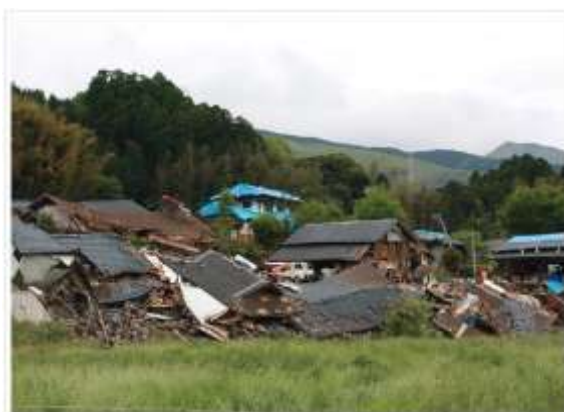
Damage in Okirihata
