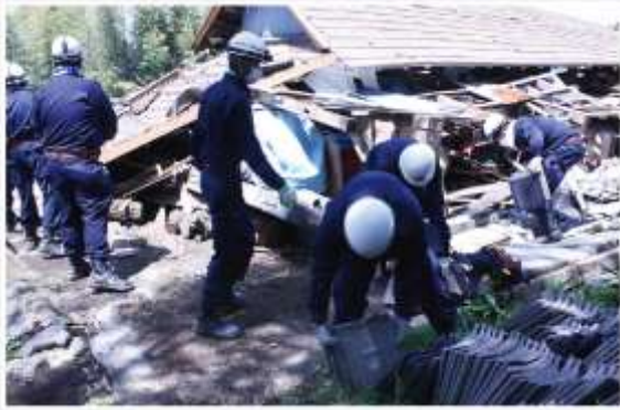
Removal of rubble
